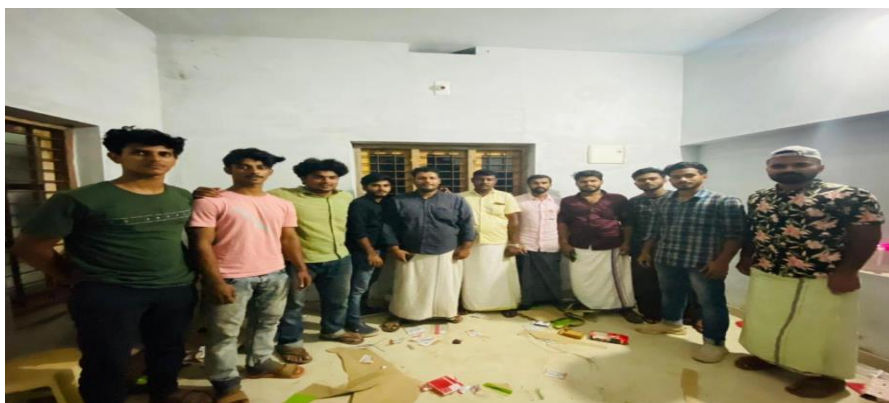
United Kattamkundu Socio Cultural Centre team who assisted in electric wiring of the house
