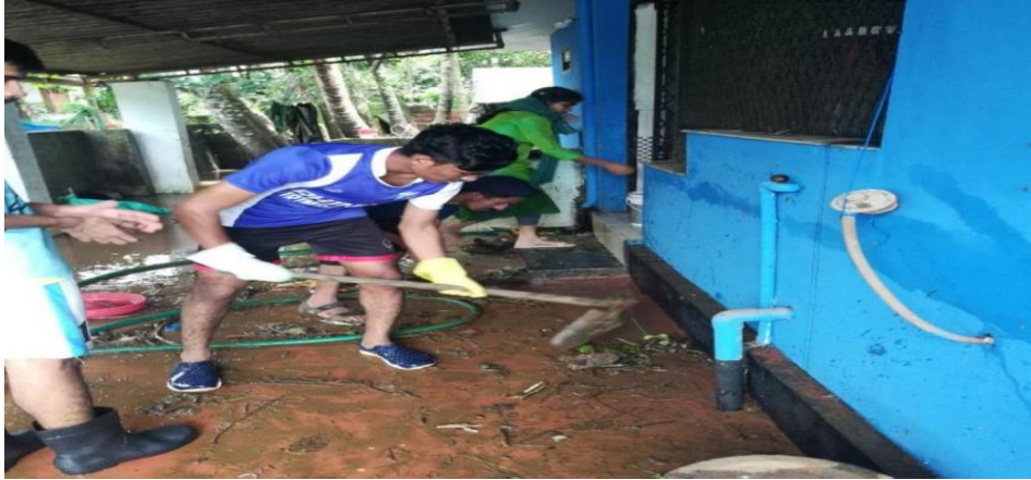
Cleaning the flood affected houses
